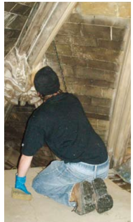
The painstaking work under way.
