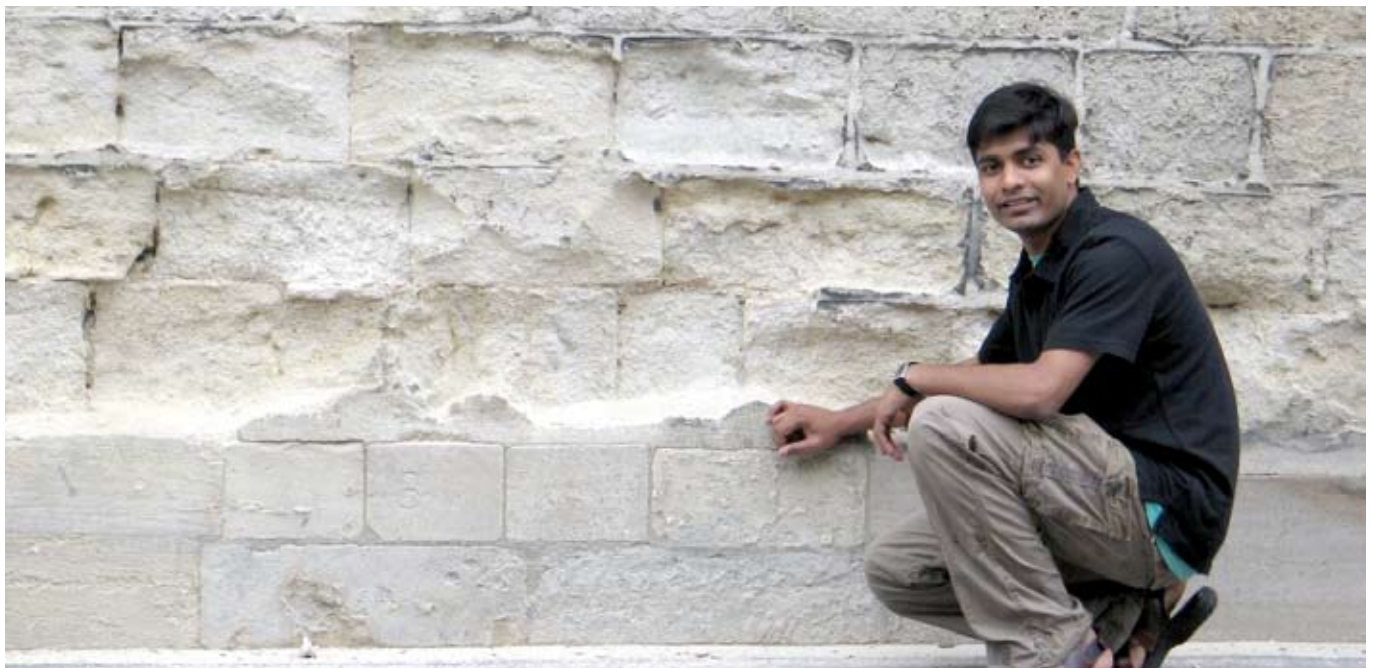
Satish surveys typical damage and decay. Note that the salt damage affects the stone at the higher level, where the salt concentration is higher.
