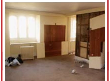
Photos by Mawuli Ladzekpo (2005, PPE)
